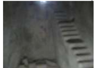
This is inside one of the massive cisterns in his palace. It would fill up during the rainy season and would supply the water for the rest of the year
