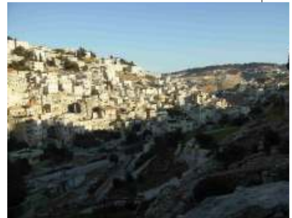
The compact buildings built today are on the exact same spots as the Biblical period. This is basically how the city of Jerusalem looked during King David's time.
